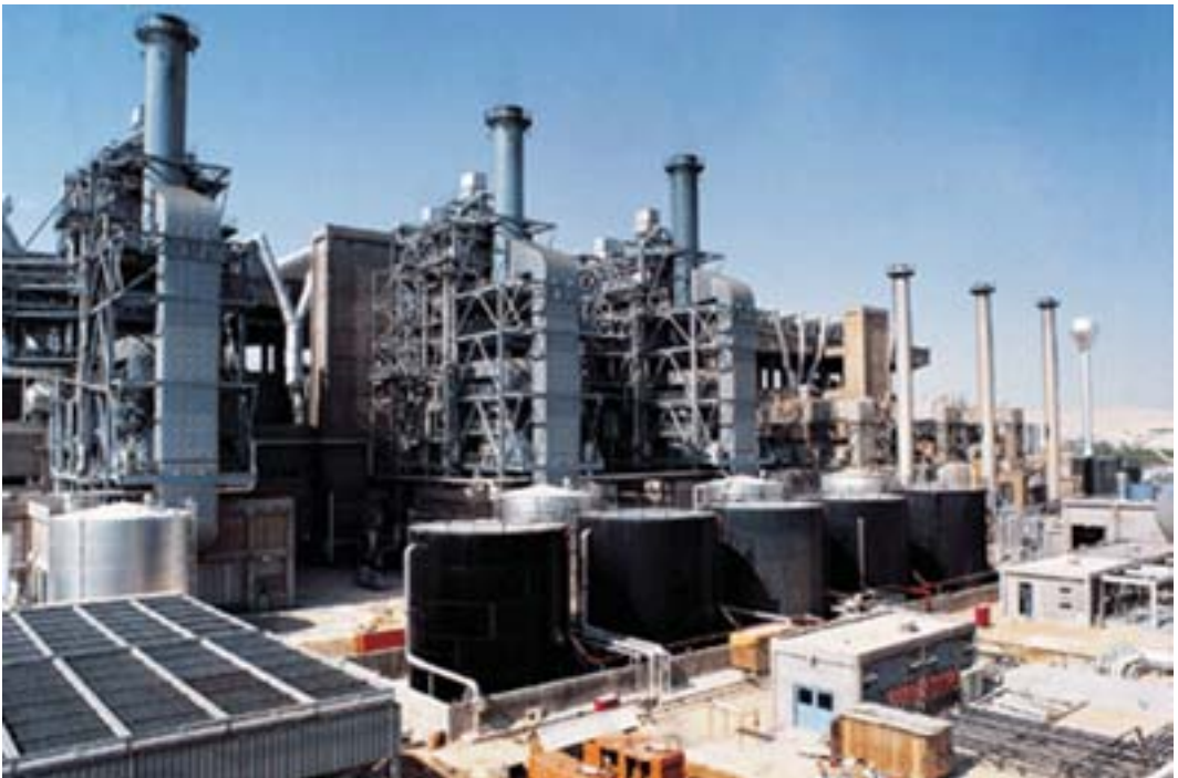
An overview of a thermal power station.
