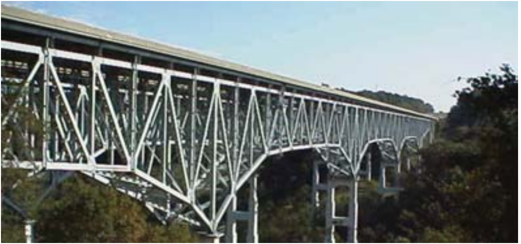
A railway bridge.
